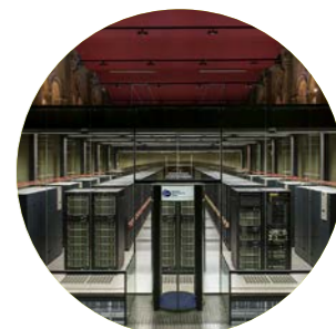
Barcelona Supercomputing Center UPC
